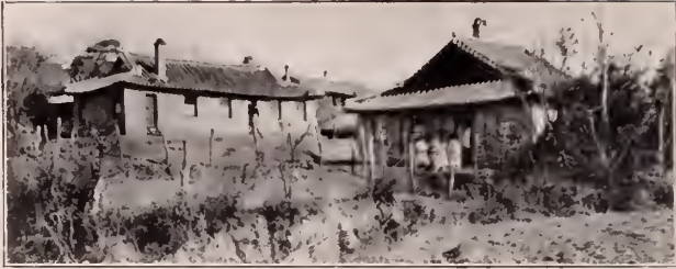
Kunsan Hospital Buildings.
